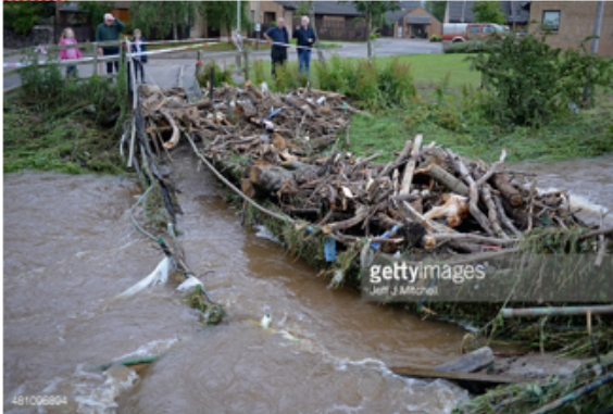
Alyth 3 – collapsed footbridge at Primary School
